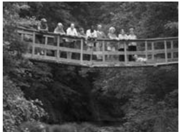
Cherry Run suspension bridge
